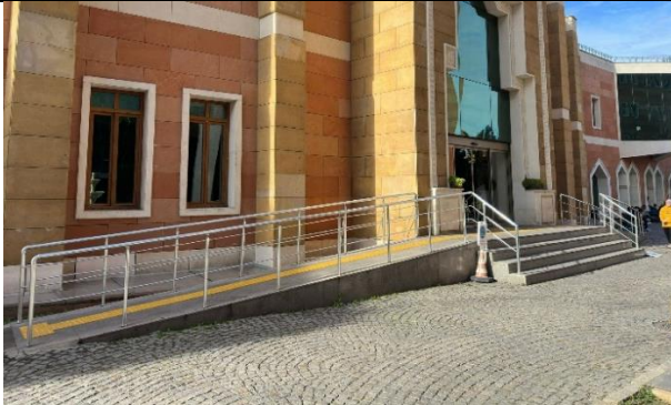
Ramps and Guiding Blocks That Have A Suitable Design for Pedestrians Having Physical Disabilities Pedestrian Paths (Yeditepe University, Turkey)
