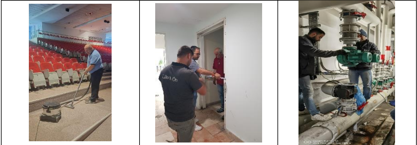
Examples of Repair and Maintenance Works
