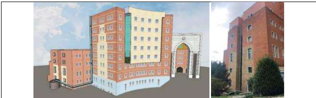
Water Conservation – Rain Water Collection (University of Yeditepe, Turkey)
