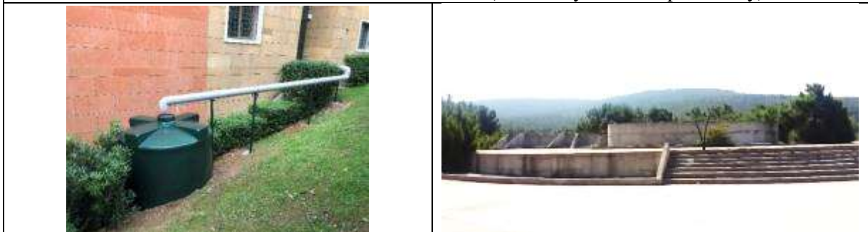
Water Conservation-Rain Water Tank (University of Yeditepe, Turkey)
