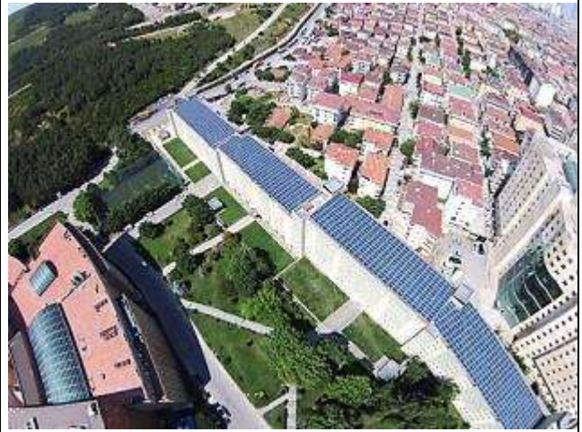
Solar Panels (Yeditepe University, Turkey)
