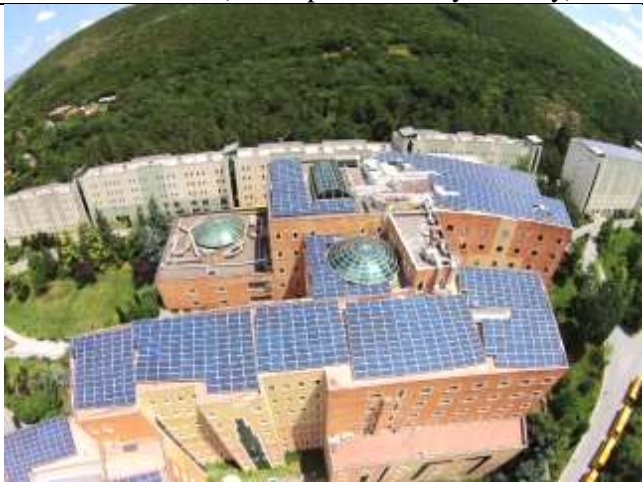
Solar Panels (Yeditepe University, Turkey)
