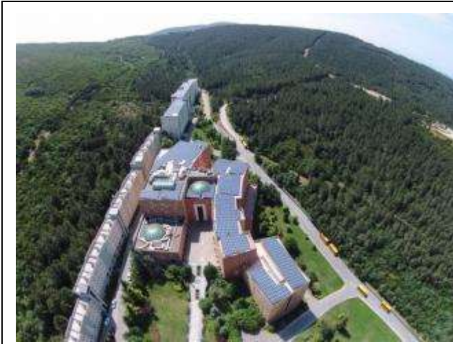
Solar Panels (Yeditepe University, Turkey)
