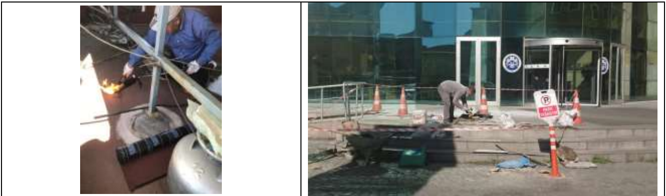
Examples of Repair and Maintenance Works
