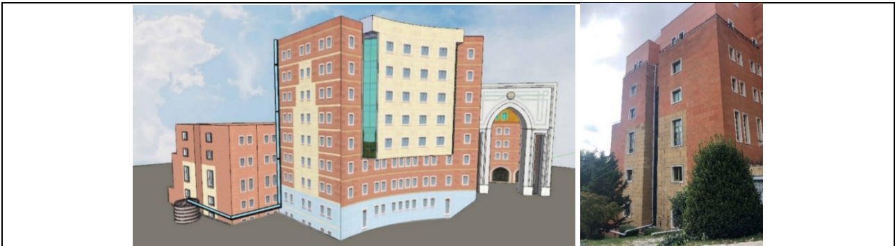
Water Conservation – Rain Water Collection (University of Yeditepe, Turkey)
