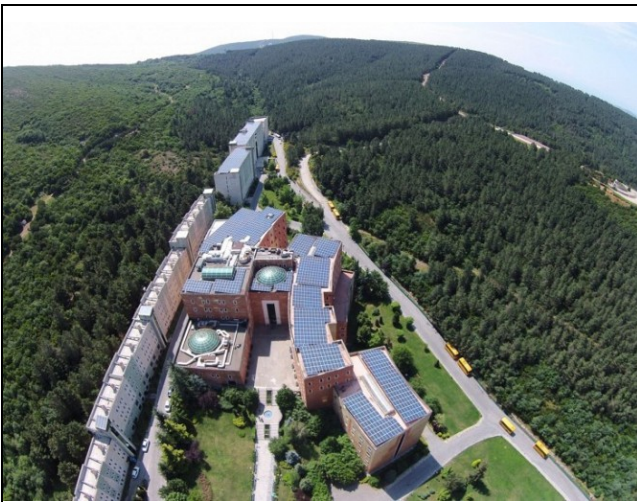
Solar Panels (Yeditepe University, Turkey)
