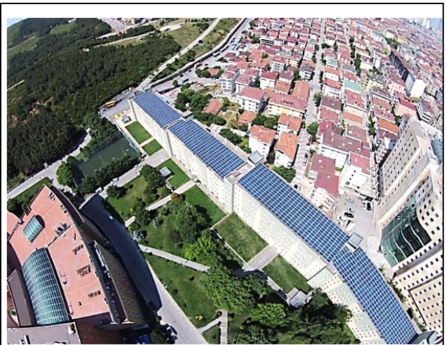
Solar Panels (Yeditepe University, Turkey)
