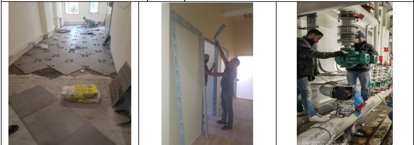
Examples of Repair and Maintenance Works
