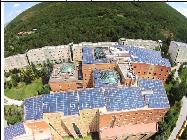
Solar Panels (Yeditepe University, Turkey)
